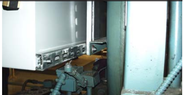
FD Motor wires routed behind the panel.
