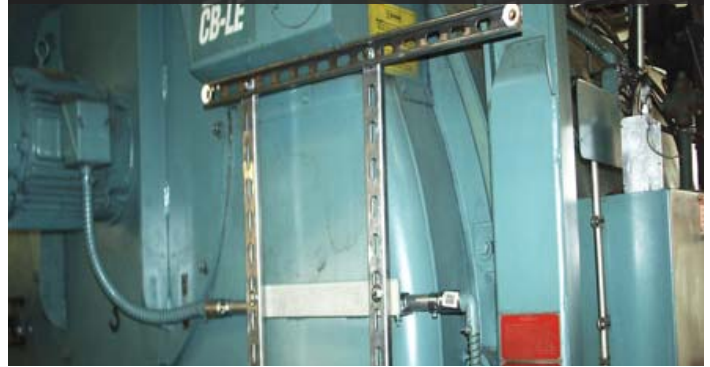
New uni-strut frame bolted to the angle supports.
