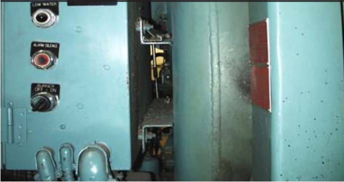
Original panel mounted to the angle supports.
