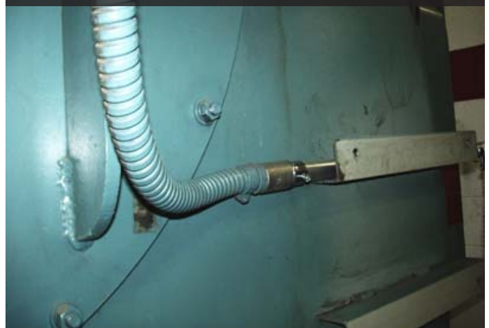
FD Motor wires routed behind the panel.
